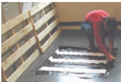
Figure 14. Modification: stapling paper strips to plastic inner roof
