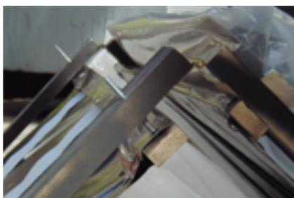
Figure 15. Modification: winding plastic inner roof around cross support and attaching to timber posts
